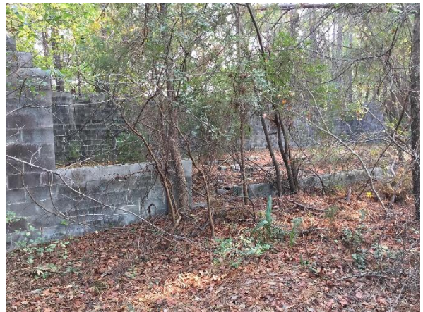
Photo #4 View of abandoned concrete block structure at approximately 1861 Clements Ferry Road.
