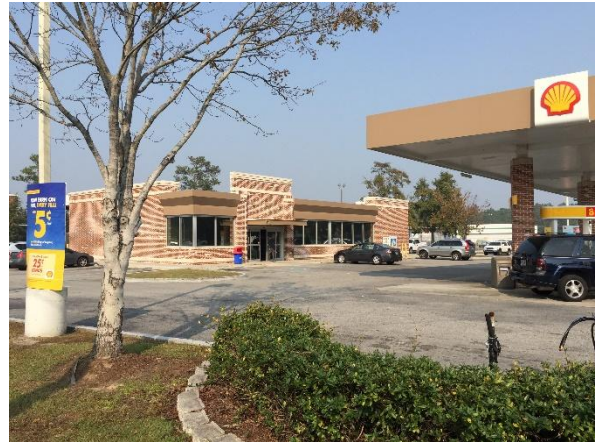
Photo #2 View of Blue Water 19 gas station at 1952 Clements Ferry Road.
